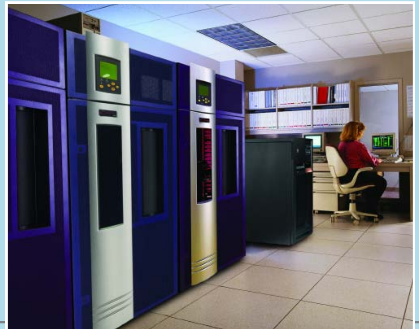
Robot/SAVE helps you manage your data center. Connect multiple System i systems to an AML and perform volume management and reporting from any system in the data center.
