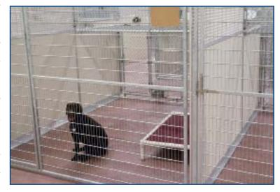
together in one large run. Since kennels are usually oriented in a row, varying the widths with a common length is the most economical and operationally efficient approach. This way, larger dogs can use a wider kennel to stretch out. Another option is to build transfer doors into the panels between kennels which can be raised to share two adjacent runs. The key is to have a variety of sizes available.
